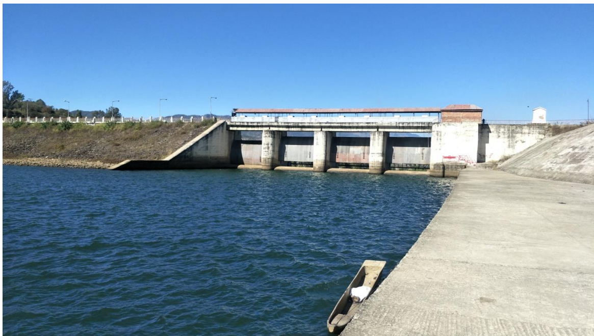
Photo 2: Spillway of Khuga dam
